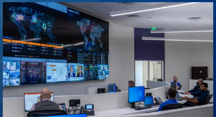
Alamo Regional Security Operations Center (ARSOC) strengthens around-the-clock collaboration between the city of San Antonio and CPS Energy information security personnel to safeguard the community's critical infrastructure against a growing threat environment.
